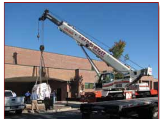
A crane lifts the new magnet required to upgrade the MRI unit.
